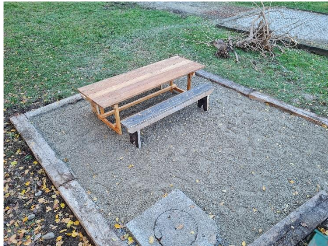
Working progress accessible path and container for disabled
