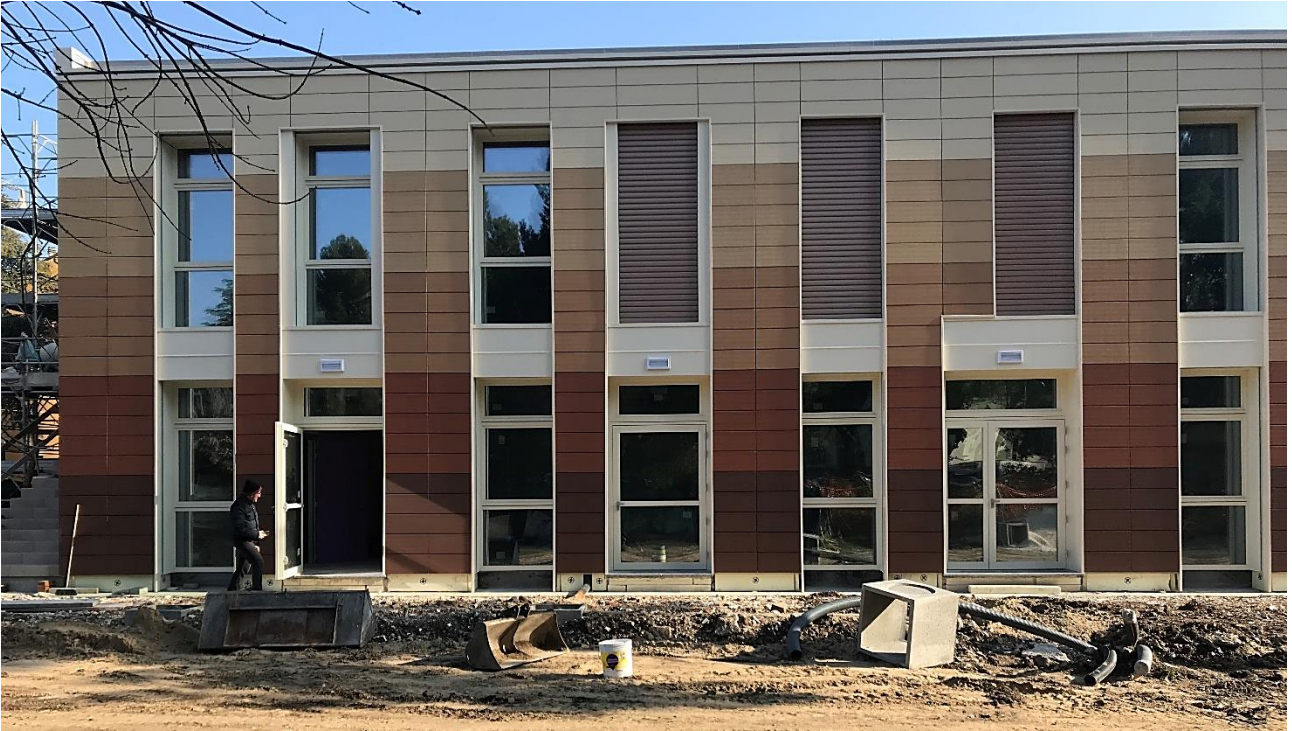
Figure 1 – Elementary/Middle School in Pesaro (Italy)
