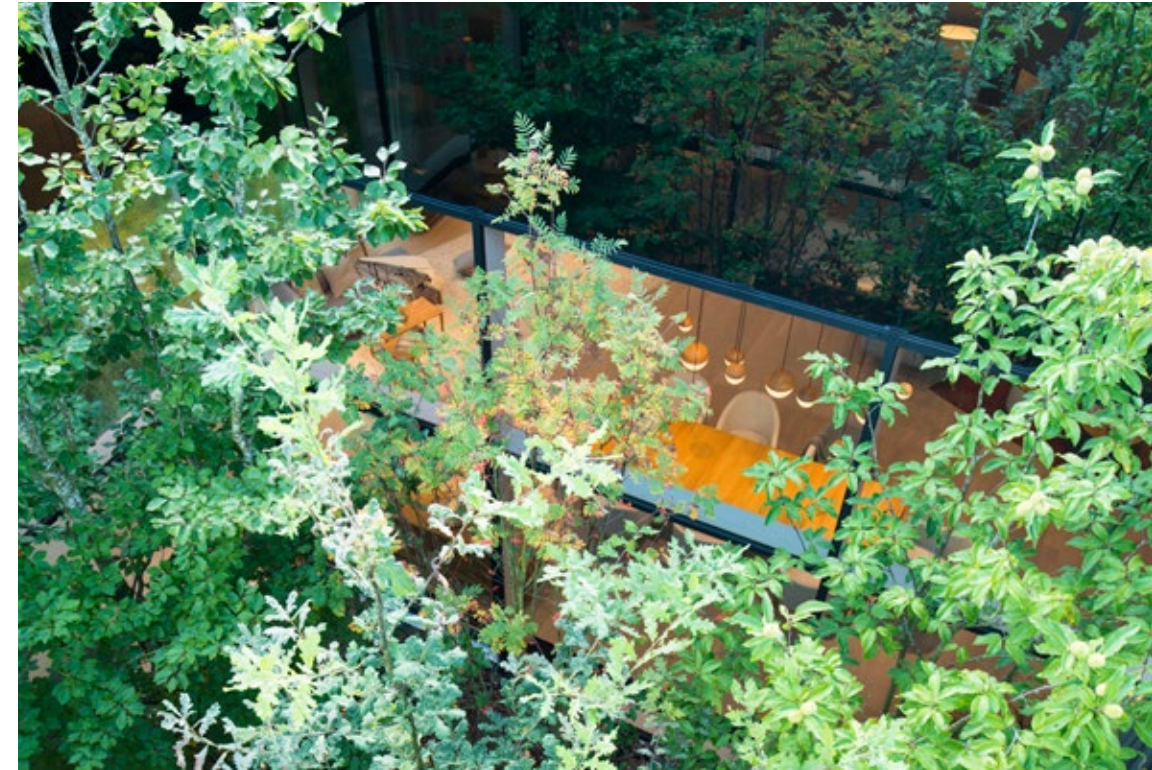
VIEW OF A BREATHING ATRIUM: Supported by active fogging on hot days, the atria actually allow the building to organically breathe in and out, cooling all interior spaces – without the use of air conditioning.
